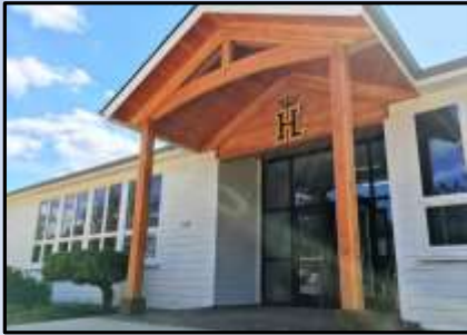
Hawthorne Elementary (Grades K-6)
